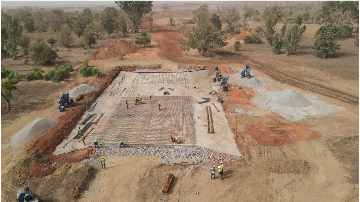
Figure 2: Nobsin River Crossing
