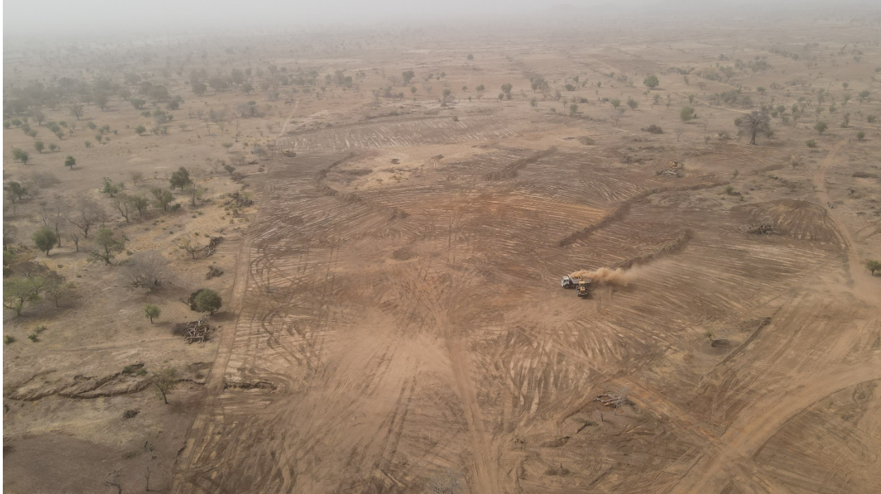
Figure 3: TSF Site Preparation
