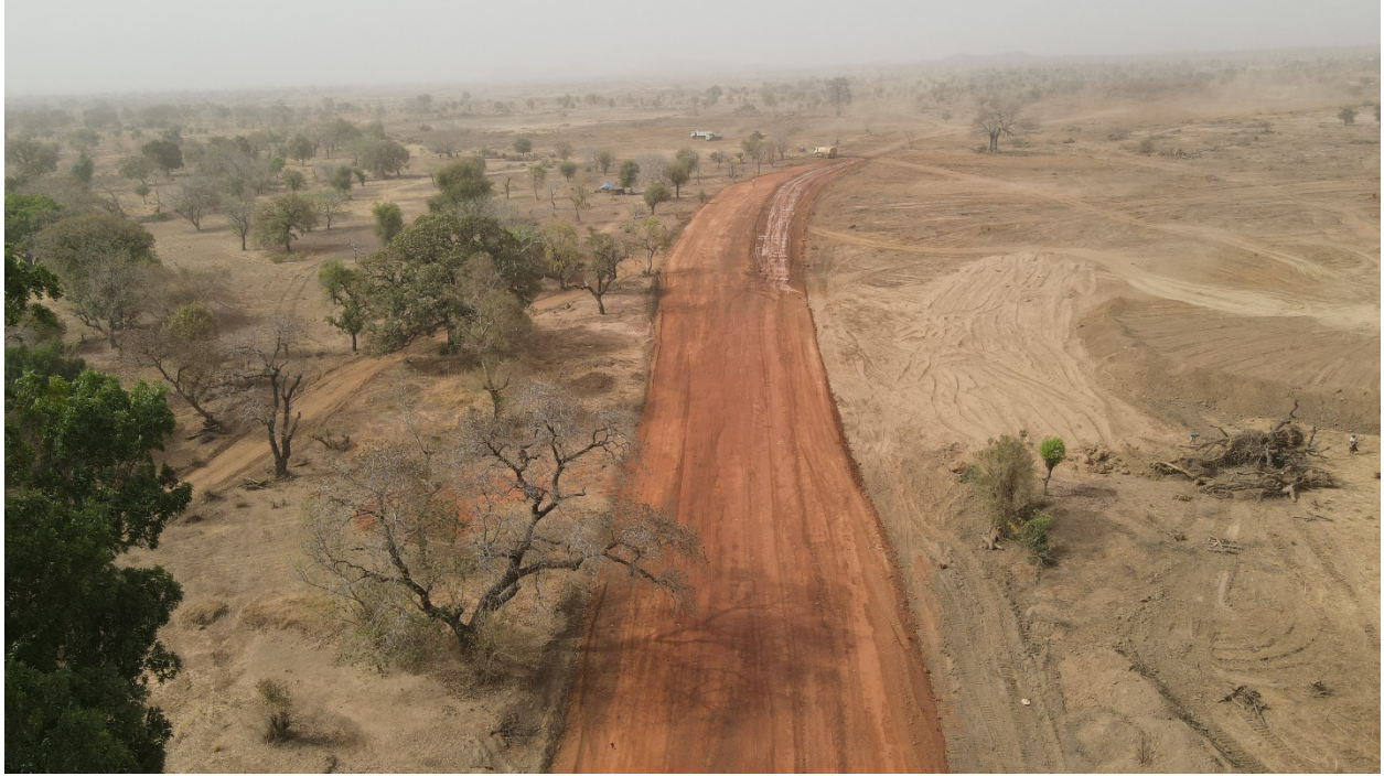
Figure 1: Site Access Road
