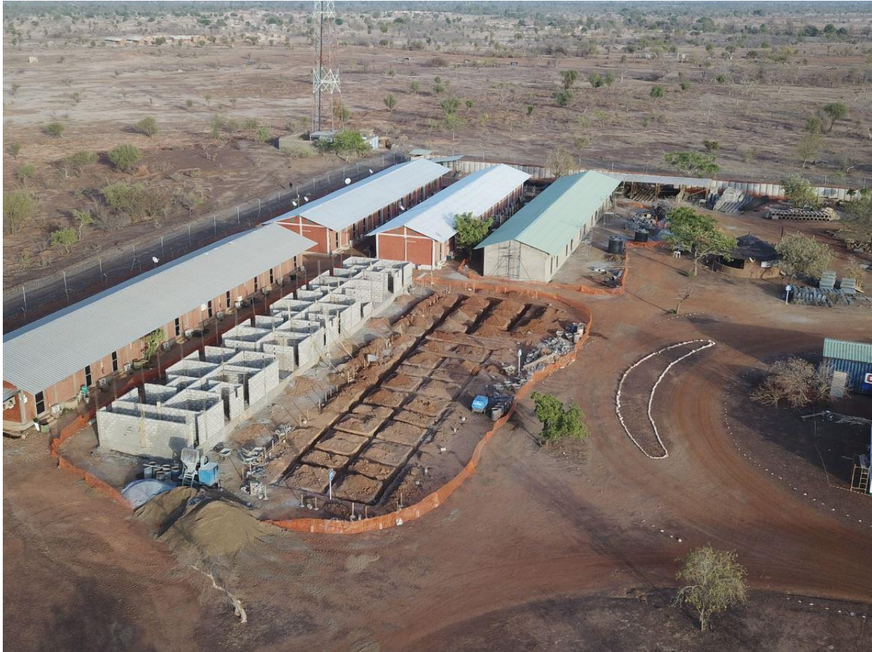
Figure 6: Camp accommodation blocks
