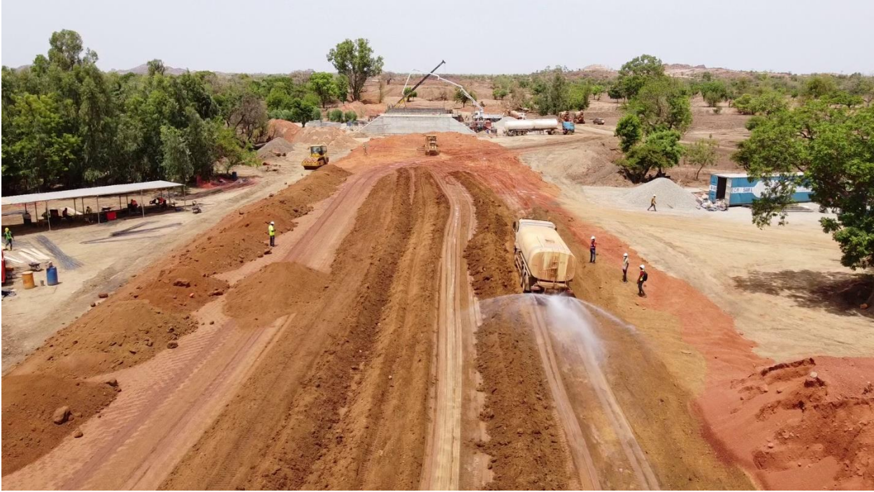
Figure 4: Main Haul Road and Nobsin River Bridge
