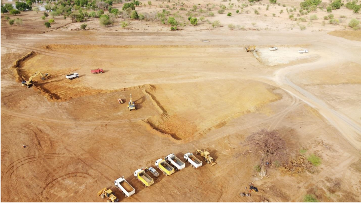
Figure 2: Construction Water Storage Facility
