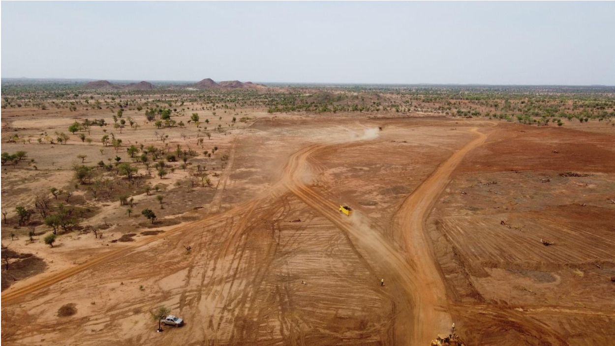
Figure 5: Process Plant Area Clearing and Grubbing
